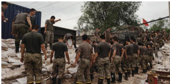
“23·7”特大暴雨期间，永定河（丰台段）封堵堵口
